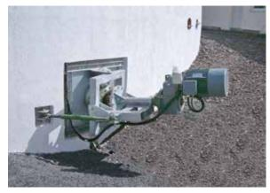
The compensator can be submerged up to 20 metres (up to 100 metres as a special version), and so the mixer can also be installed at the bottom of any tank. The corresponding installation components can be manufactured.
